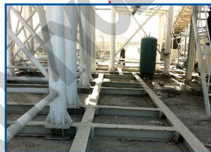
水泥仓整体钢底盘 Cement silo steel whole chassis
